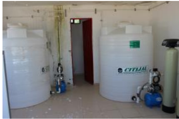
Photo 14. Abandoned purification plant in the community of 'El Zancarrón' in Santo Domingo.
