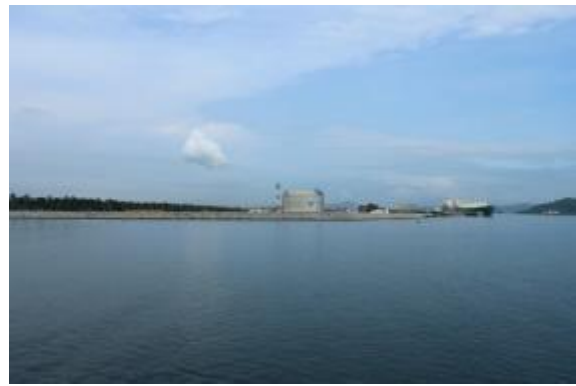
Photo 6. Liquefied Natural Gas Terminal.
