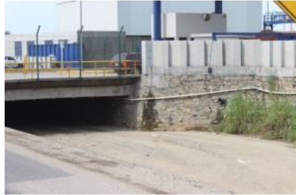
Photo 12. Drainage from storage yards to a channel.
