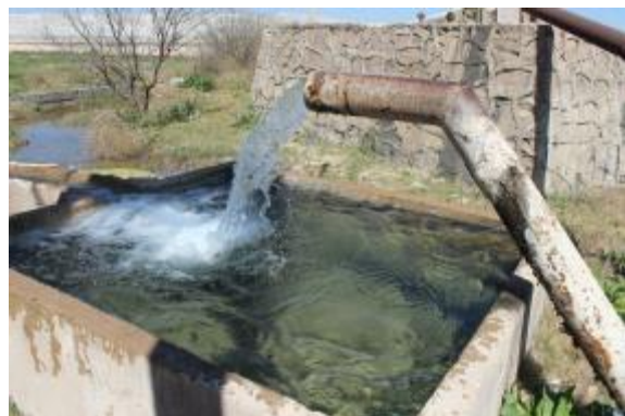
Photo 18. Water well for agriculture in the community of 'El Mezquite' at Villa de Arista.
