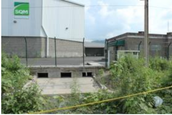
Photo 9. Drainage from storage yards to the street.
