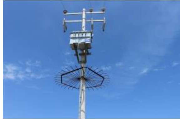
Photo 26. Protection infrastructure for electrical transformers of a water well to prevent robbery in Villa Hidalgo.
