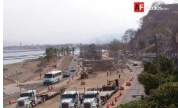
Image 4. Road distributor in Manzanillo linked to the tunnel for connection to railroad deviation.
