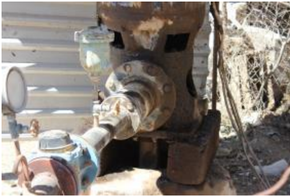
Photo 19. Status of an old pump for a well in the community of 'San José del Arbolito' in Villa de Arista.
