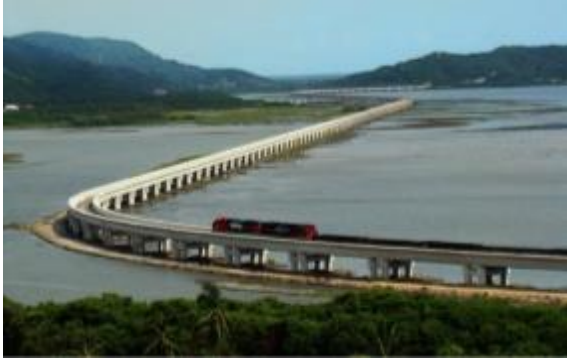
Image 1. Railroad deviation within the coastal lagoon.
