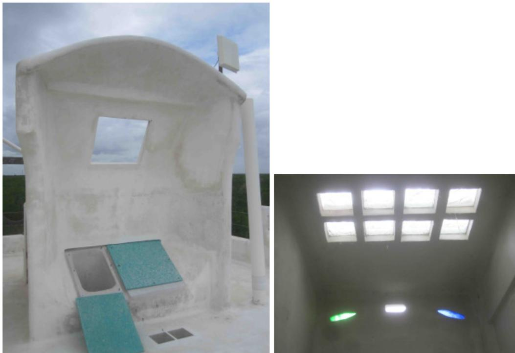
Figure 9-2: Wind deflector with vent ducts (left), natural lighting in El Arca. Pictures taken by Moie, 2012
