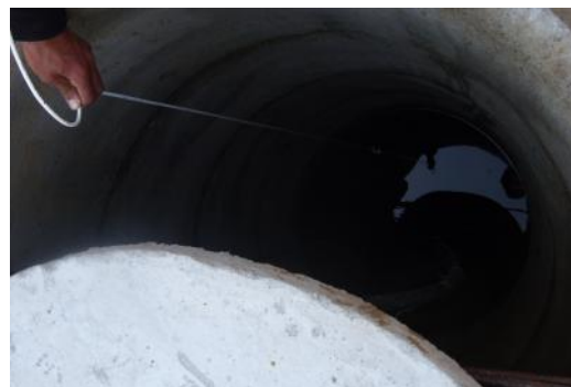
(b) Dug water well is handmade with a higher diameter and a cover of concrete. The water is extracted with a pump.
