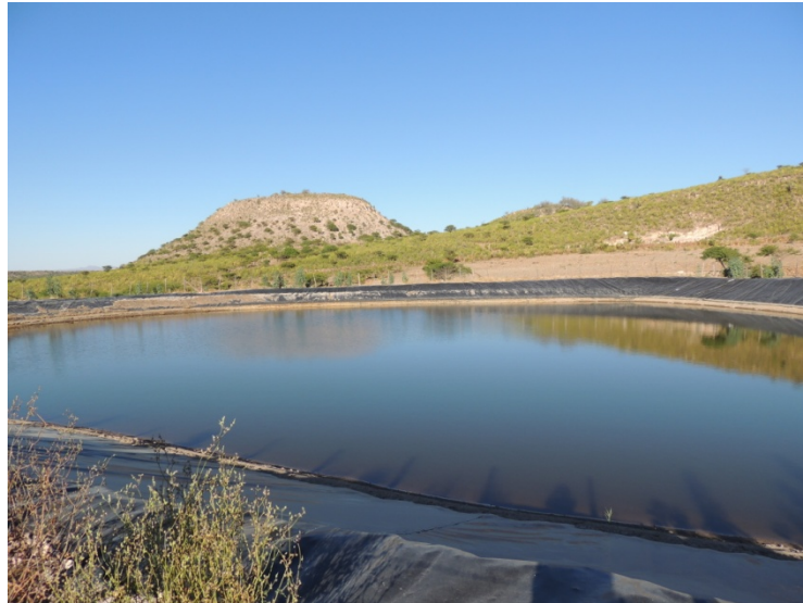
Figure 23: Water collector Santiago Bayacora in Durango, Pronatura México 2014
