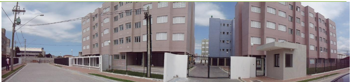
Figure 4.9: Fence and Security Checkpoint. 427
