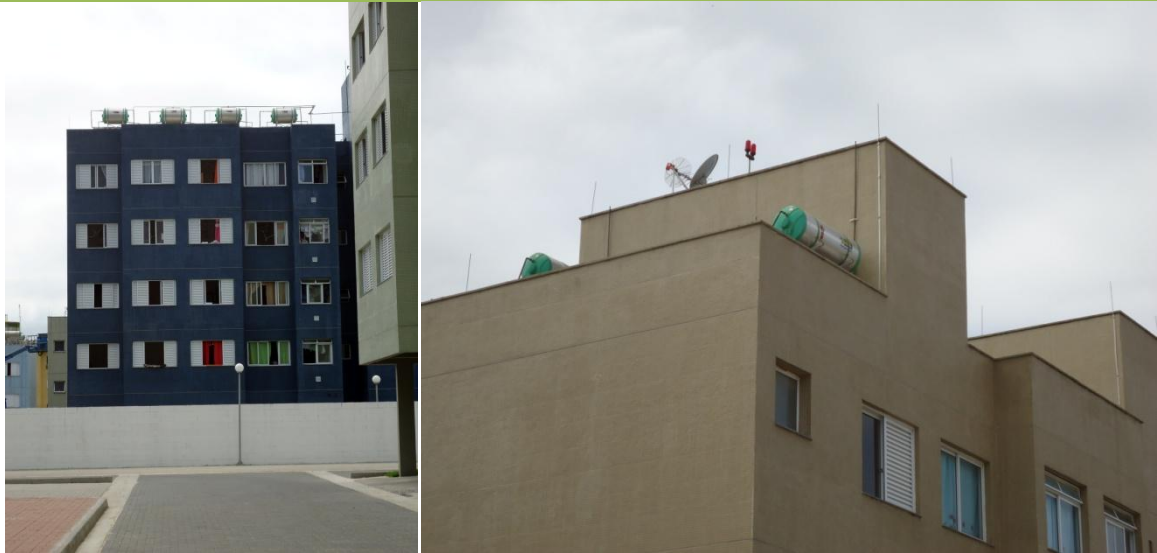
Figure 4.10: Solar Water Heaters. 428
