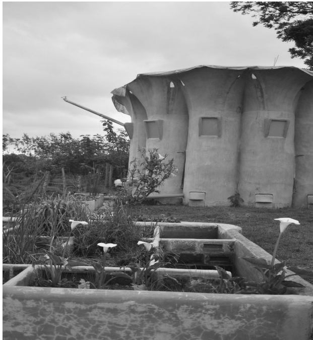
Figure 15: Gray water recycling, Las Cañadas
