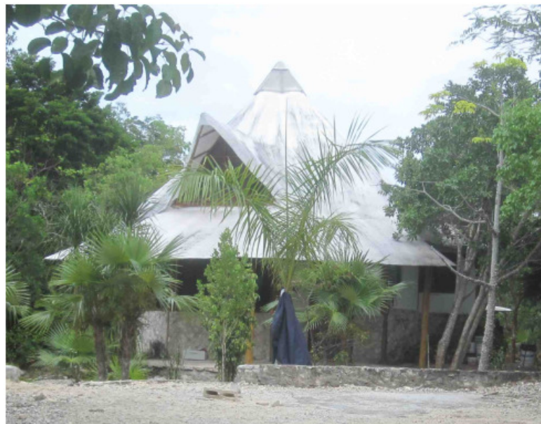
Figure 9-6: Ferrocement roof (reinforced concrete), Puerto Morelos. Picture taken by Moie, 2012
