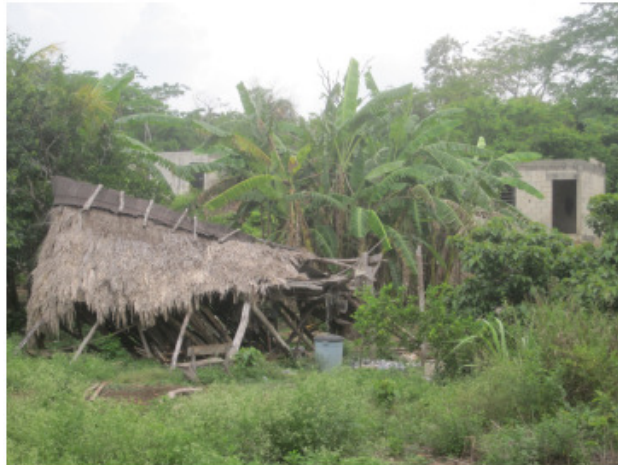
Figure 8-2: Damage after hurricane Wilma and recent trends in San Román. Picture taken by Moie, 2012
