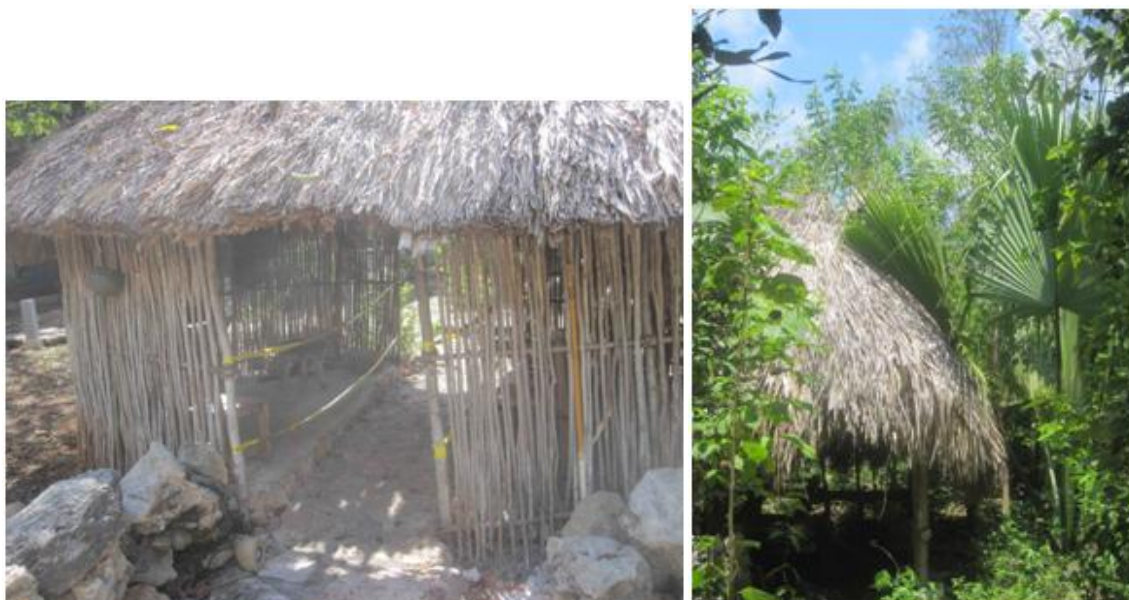
Figure 4-4: Model of a traditional Maya house (left); roof of fan palm (huano) next to growing fan palm. Pictures taken by Moie, 2012
