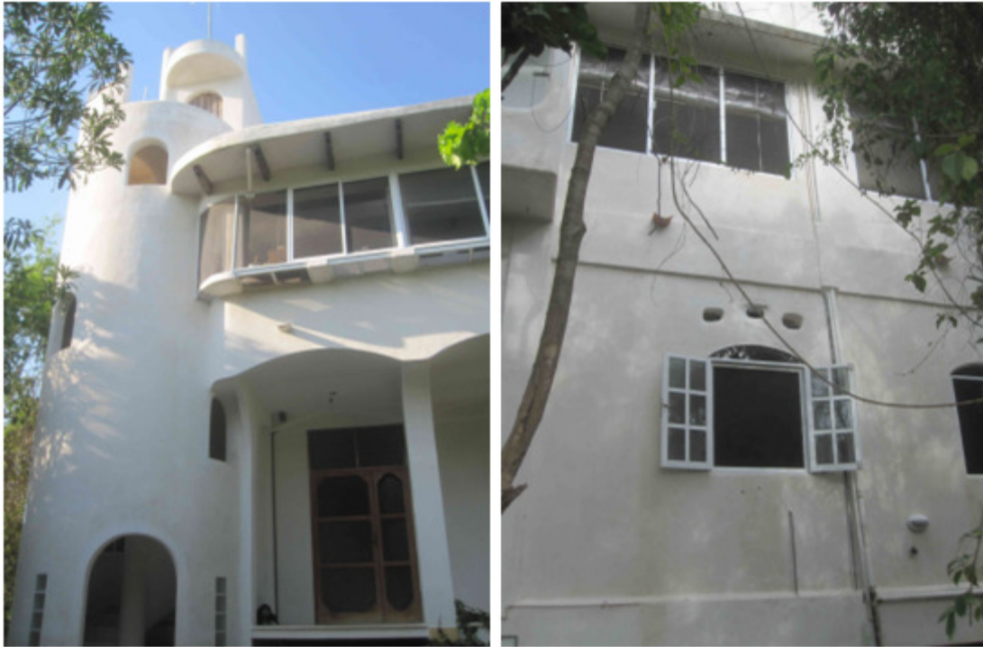
Figure 9-1: El Arca from south view (left) and the west facade. Pictures taken by Moie, 2012
