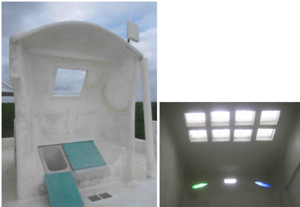
Figure 9-2: Wind deflector with vent ducts (left), natural lighting in El Arca. Pictures taken by Moie, 2012
