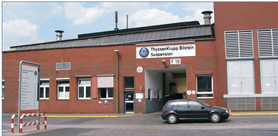
Figure 4.8 Front entrance of TK-Hagen industrial plant (Photo: ISGUS GmbH, 2008).
