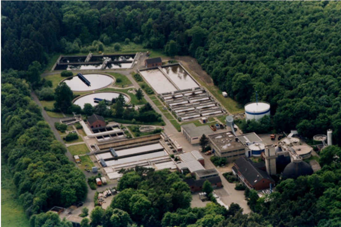
Figure 1. Beningsfeld Waste Water Treatment Plant
