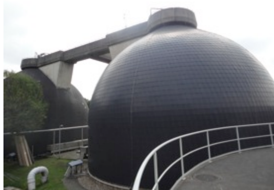
Figure 3. Anaerobic Digestors 1 and 2
