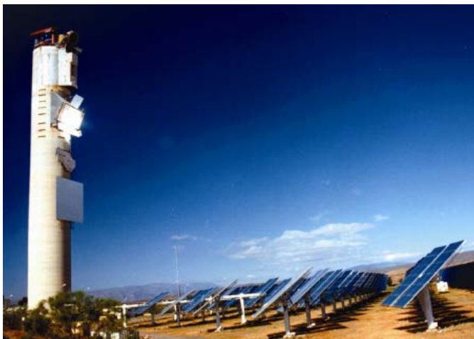
Picture 3: Heliostat Field: Solar Tower CESA-I Source: (Ciemat, 2010)
