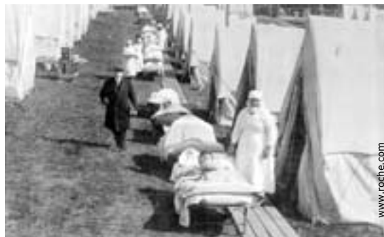
Hospital de emergencia, Brookline, Massachusets, USA. 1918.
