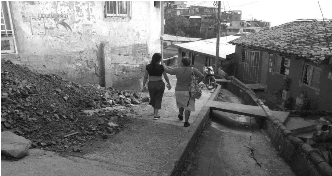
Figure 45. Obstacles and no railings or protective signage in sidewalks. Taken from transect walk activity on April 2022
