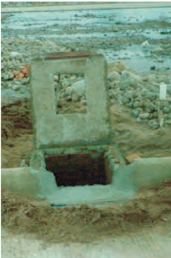
Sewer grate | Boca de tormenta
