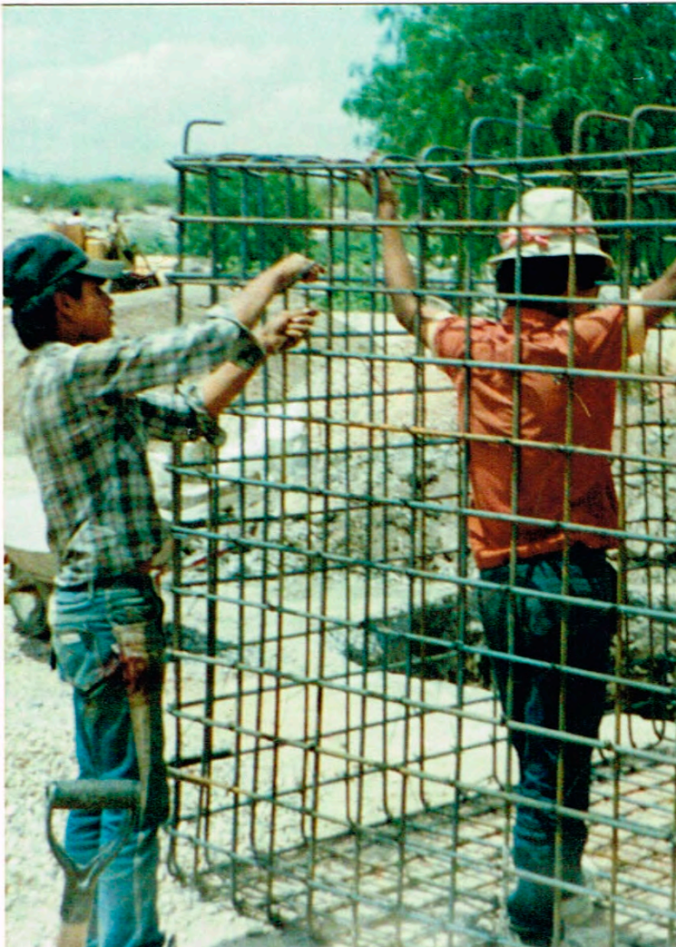
Streetlight reflectors' supporting steel structure | Estructura de acero para bases de reflectores
