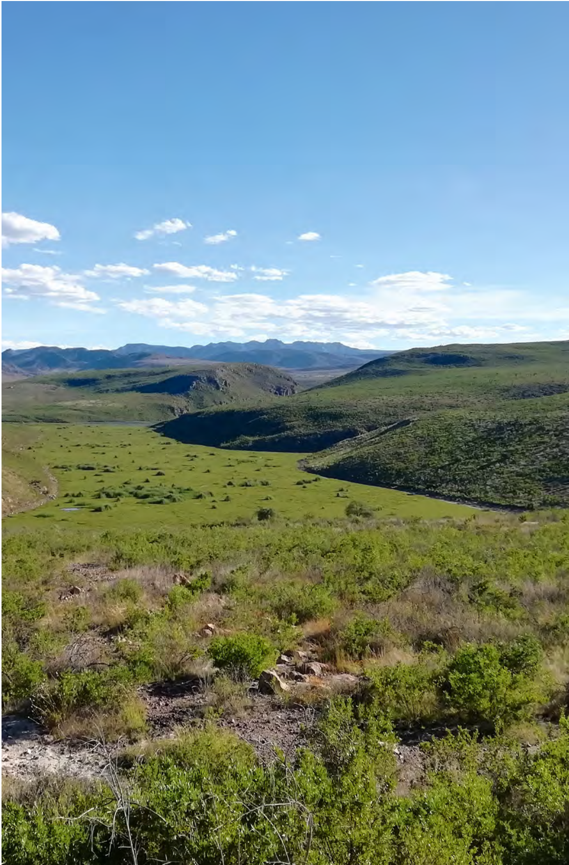
San Jose dam reservoir basin covered by water Hyacinth | Cuenca de la presa San José cubierta de lirio
