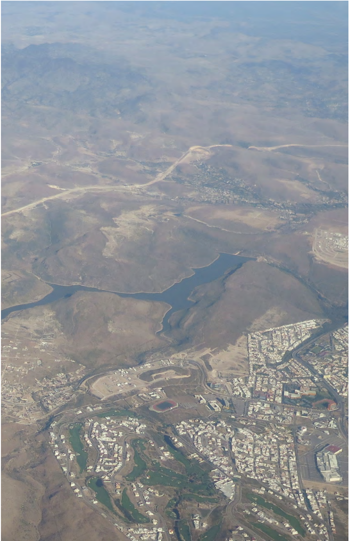
San Jose dam's aerial view | Vista aérea de la presa San José
