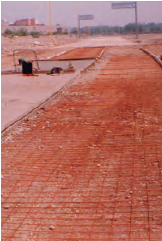
Concret cast | Colado de concreto
