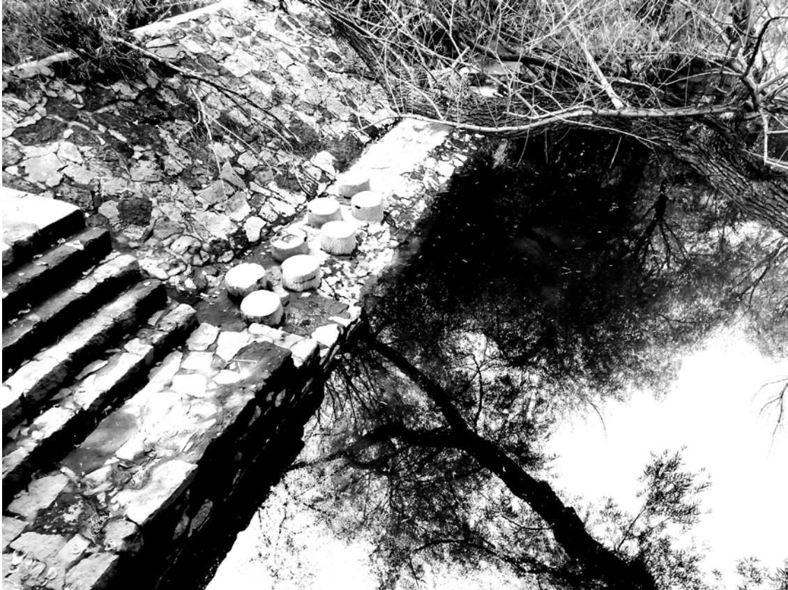
San Jose dam | Presa San José
