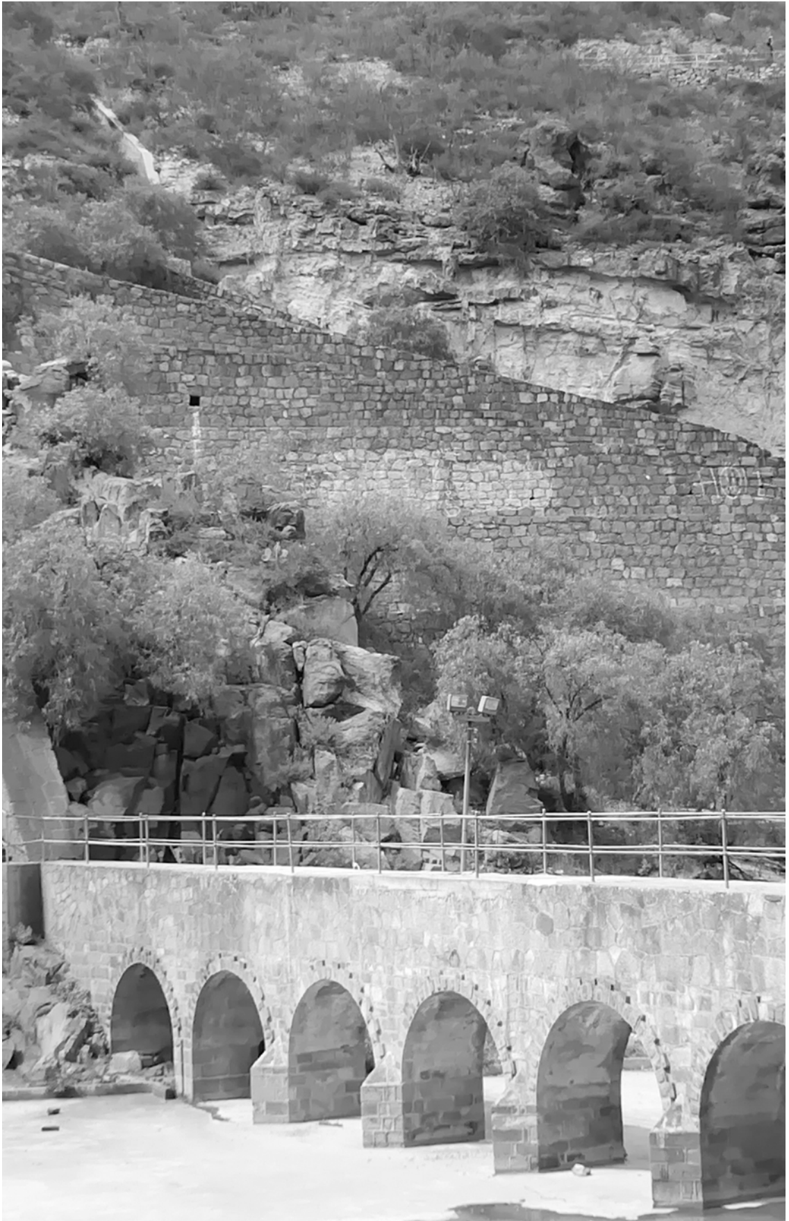
San Jose dam | Presa San José
