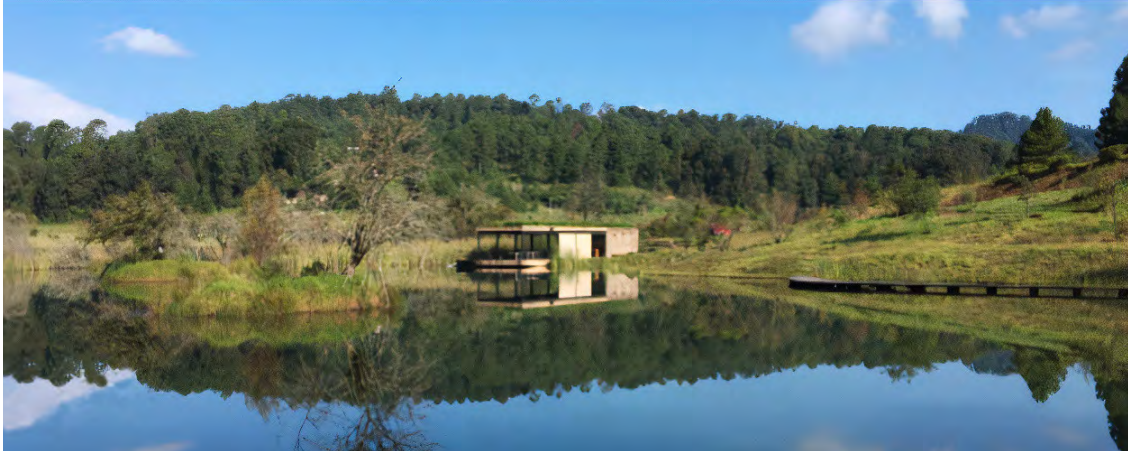
Lower lake with communal facility | Lago inferior con instalaciones comunes
